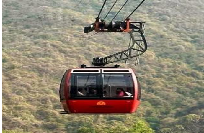
TIMBER TRAIL ROPEWAY PARWANOO
